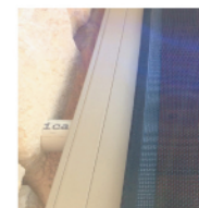
Exterior Rated Pipe used for Spacing Track
